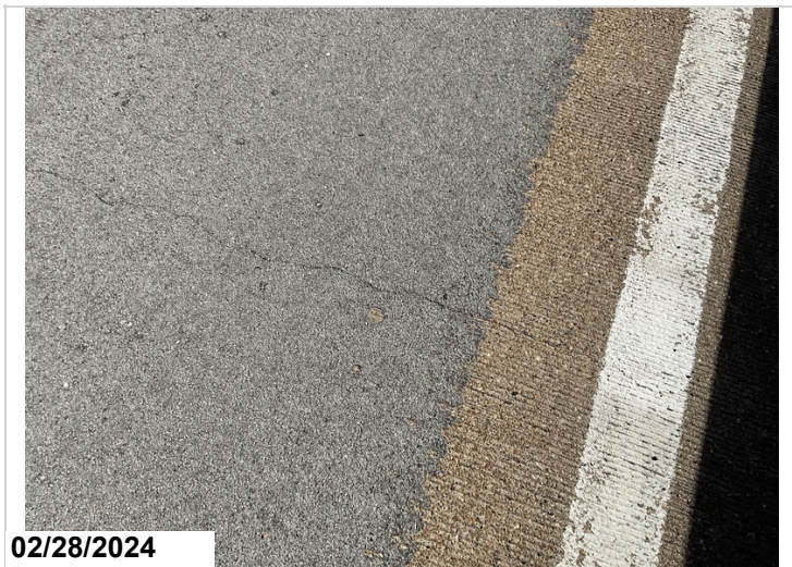
Typical deck crack
