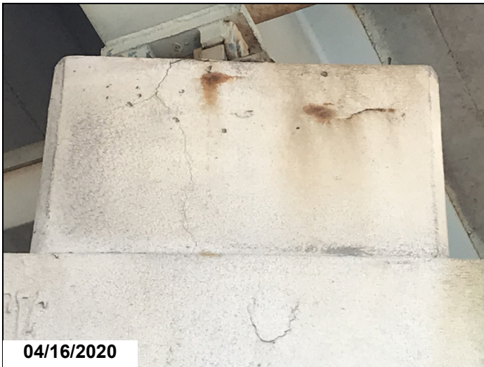
Typical cracked riser under bearing
