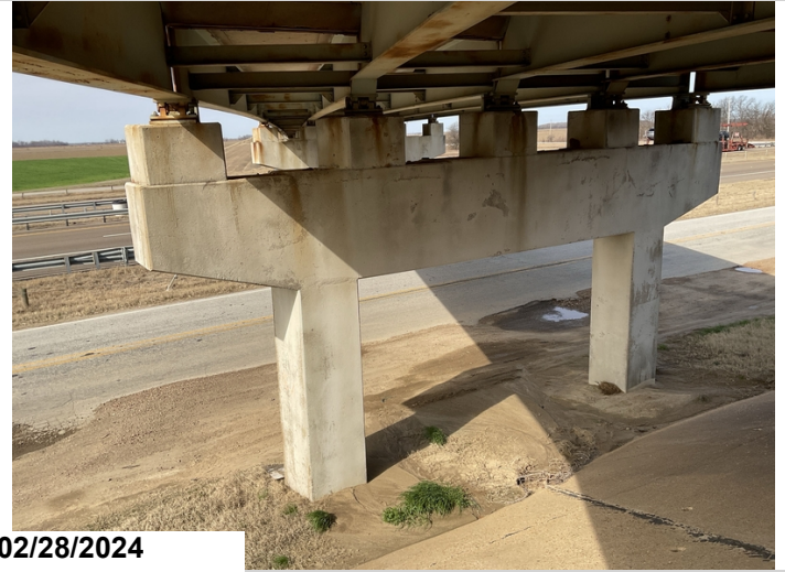
Bent 6, Pier Cap, Ahead: Vertical cracks under girders 1, 2, 5, risers, riser under girder 3 is spalled at top, and riser under girder 4 has cracking with rust staining. 3LF CS2, 1LF CS3, 1LF CS3
