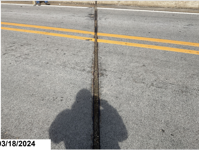
Bent 3, Compression Joint Seal: 14' of lost adhesion seal is sagging. 14LF CS3
