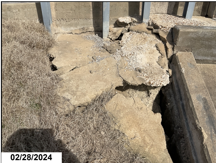
Abutment 1, Approach Roadway & Shoulder, Right: Large void under roadway with a failed old repair.
