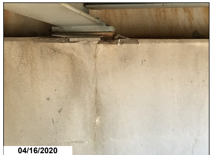
Abutment #2 typical spall and vertical crack under bearing
