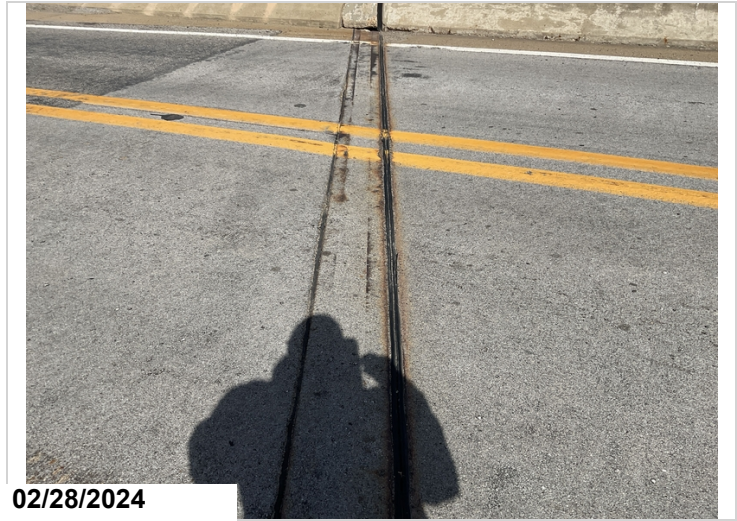
All Joints, Compression Joint Seals: Weathered and cracked. 144LF CS2
