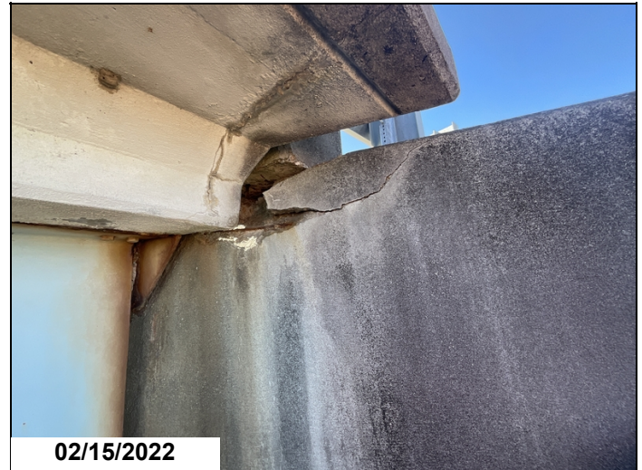
Abutment #1 left wing spalled at top with exposed rebar
