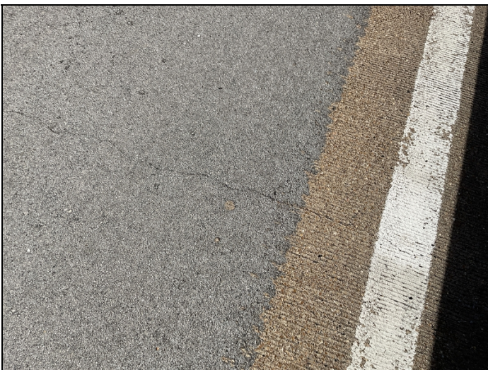
Typical deck crack
