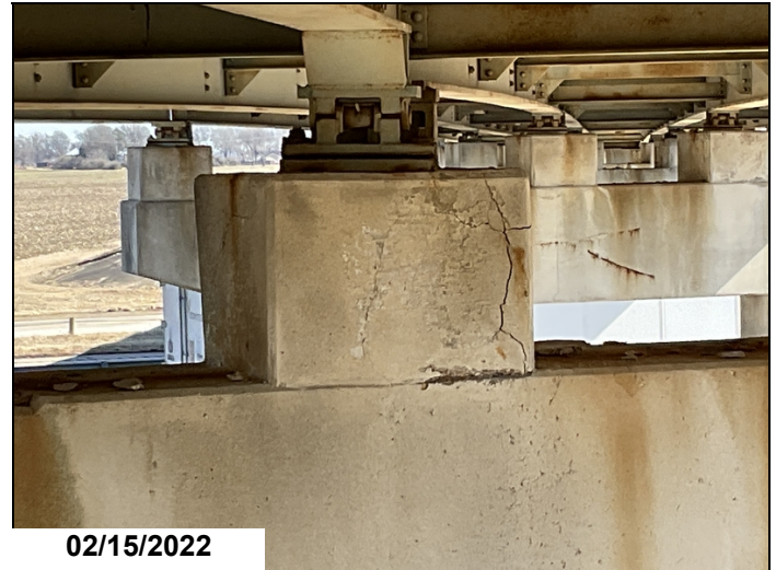
Bent #2 riser under girder #3 cracked and delaminated
