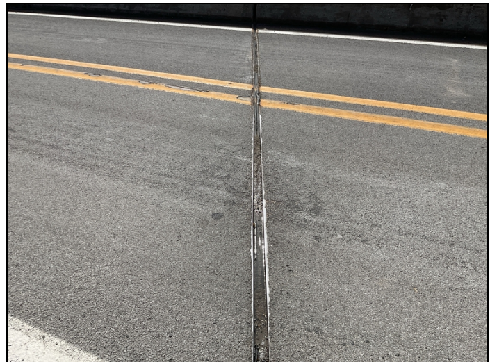
Bent 6, Compression Joint Seal: 10' of lost adhesion seal is sagging. 10LF CS3
