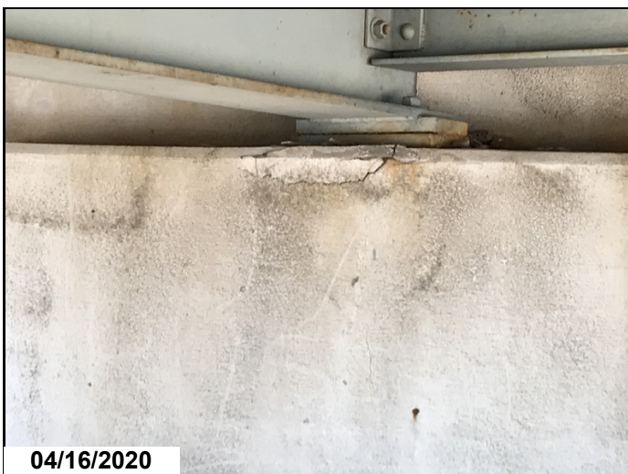
Typical delaminated area, crack, spalled area under bearings abutment #1.
