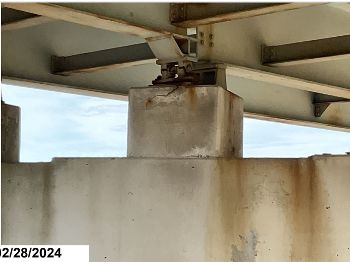
Bent 2, Pier Cap, Back, Under girder 2: 1' spall with exposed reinforcing steel. Reinforcing steel has no section loss. 1LF CS2
