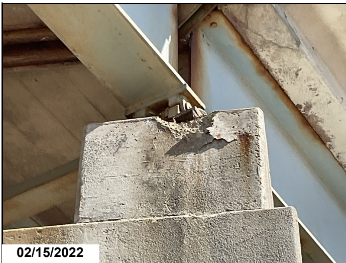
Bent #3 cap back face riser under girder #5 spalled at t
