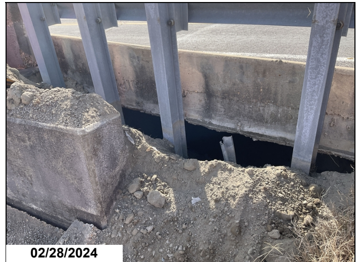
Abutment 1, Approach Roadway & Shoulder, Left: Large void 5' (depth) under roadway.
