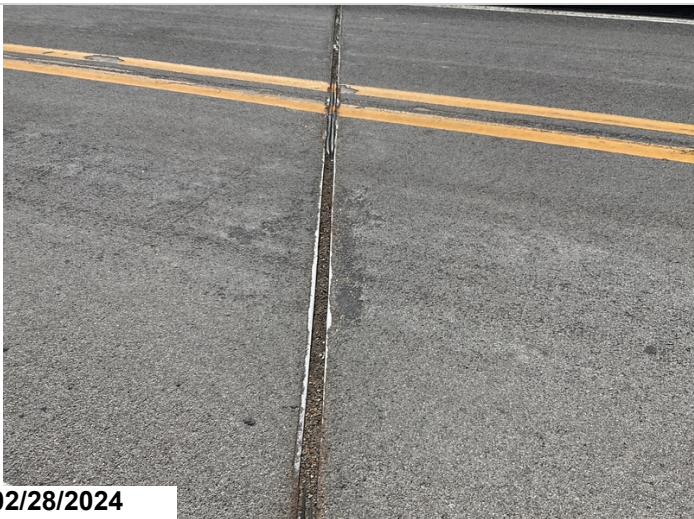
Bent 4, Compression Joint Seal: 18' of lost adhesion seal is sagging. 18LF CS3
