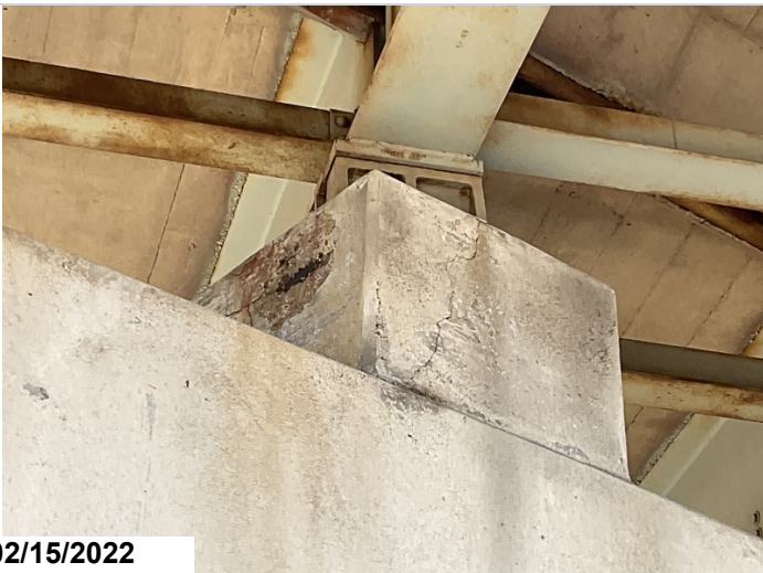
Bent 3, Pier Cap, Back, Under girder 3: Riser spalled with exposed reinforcing steel. Reinforcing steel has moderate section loss.
