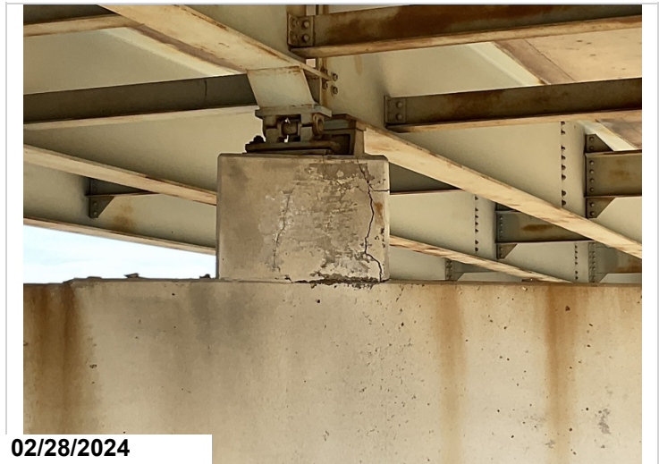
Bent 2, Pier Cap, Back, Under girder 3: 1' spall with exposed reinforcing steel. Reinforcing steel has no section loss. 1LF CS2
