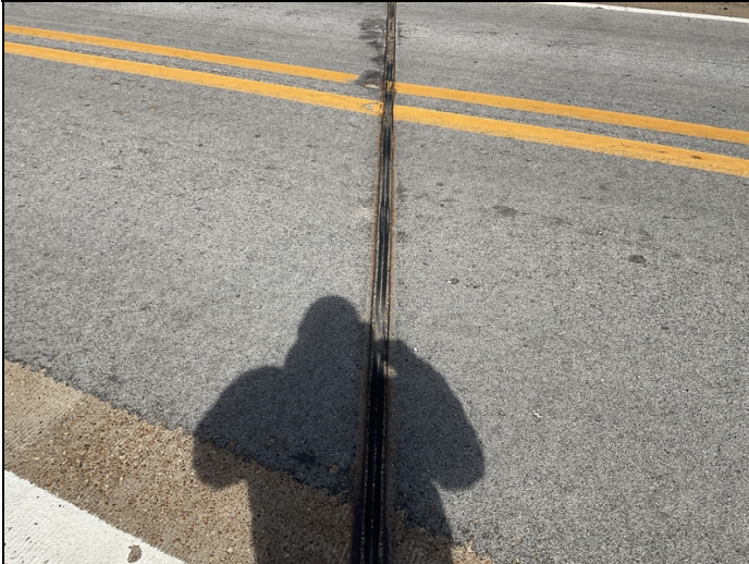
Bent 2, Compression Joint Seal: 7' of lost adhesion seal is sagging. 7LF CS3
