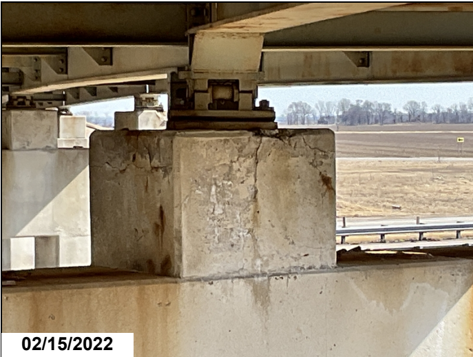
Bent #2 riser under girder #4 cracked and delaminated
