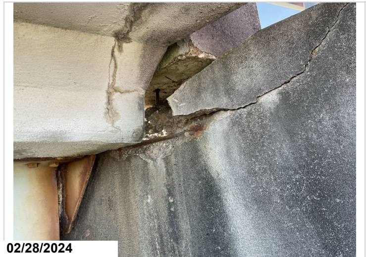
Abutment 1, Left, Top: Spalled exposed reinforcing steel. Reinforcing steel has minor section loss. 2LF CS3
