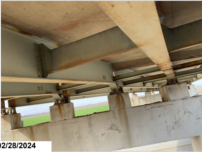
All Spans, All Girders, Full Length: Paint is discolored and oxidized with minor areas of bare steel full length. 6,445SF CS2, 6,446SF CS3, 678SF CS4
