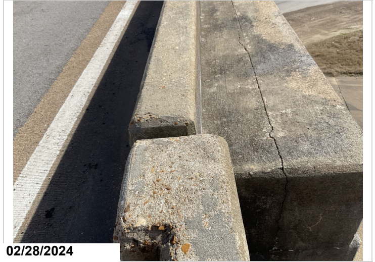
Bring rail extension crack full length of structure
