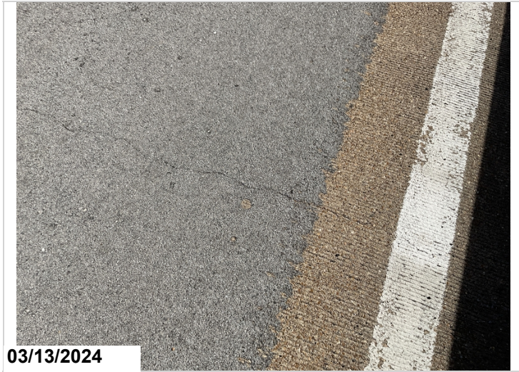
Typical deck crack
