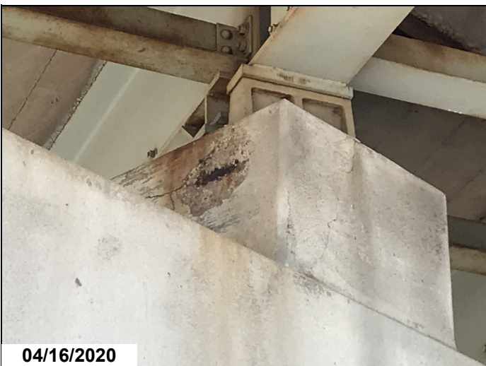
Bent #2 under girder #3 right side has one foot spall exposed rebar.
