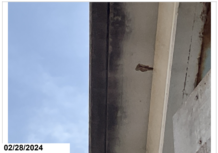
Deck Undersurface Overhang, Left, 4' From Bent 4: 8" spall with exposed reinforcing steel. Reinforcing steel has minor section loss. 1SF CS3
