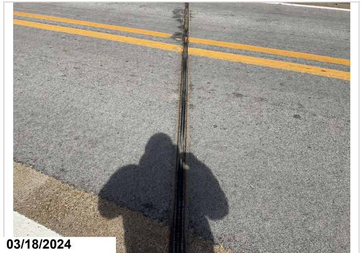
Bent 2, Compression Joint Seal: 7' of lost adhesion seal is sagging. 7LF CS3
