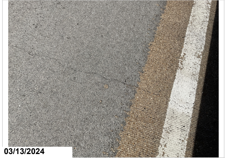
Typical deck crack
