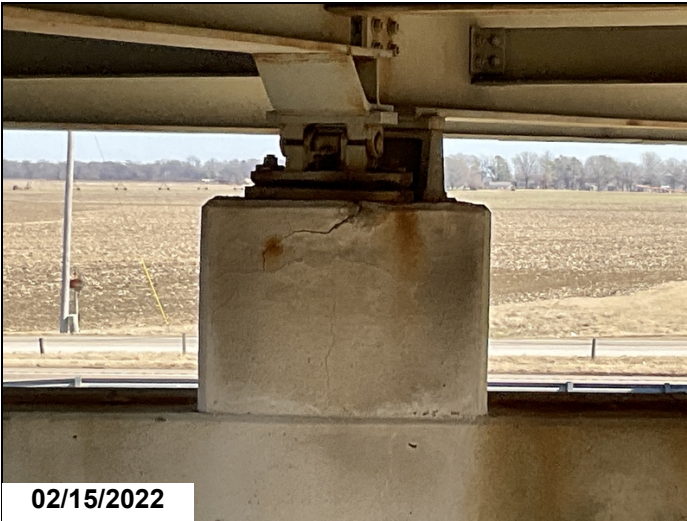
Bent #2 riser under girder #2 cracked and delaminated
