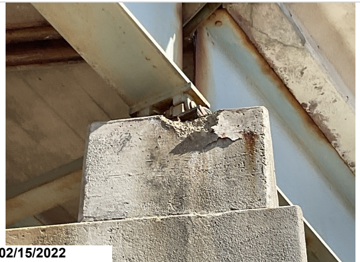
Bent 3, Pier Cap, Back, Under girder 5: Riser spalled at top no exposed reinforcing steel. 1LF CS3
