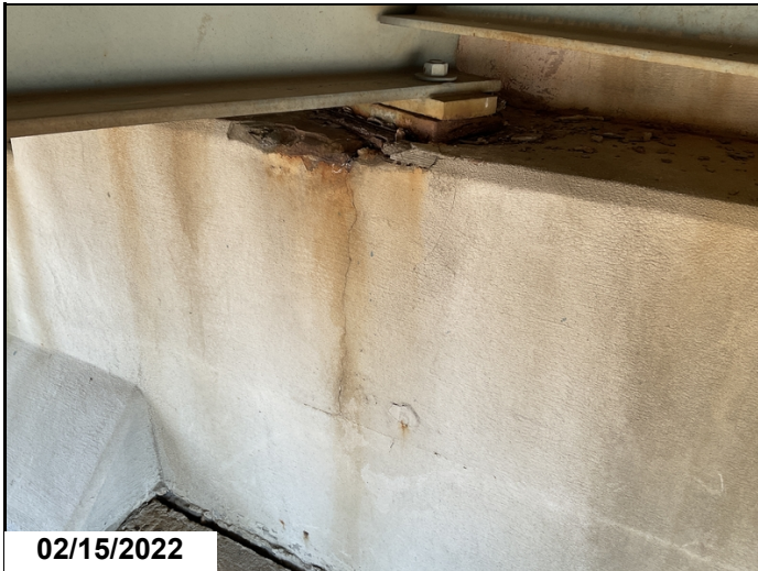
Typical vertical crack and spall under abutment bearing.
