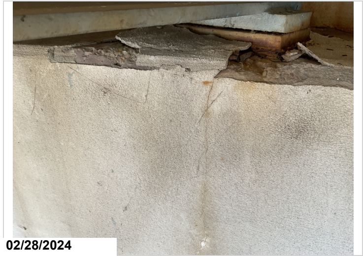
Both Abutments, Pile Caps, Top, Under Bearings: Spalled no exposed reinforcing steel. 6LF CS3
