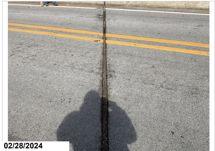
Bent 3, Compression Joint Seal: 14' of lost adhesion seal is sagging. 14LF CS3
