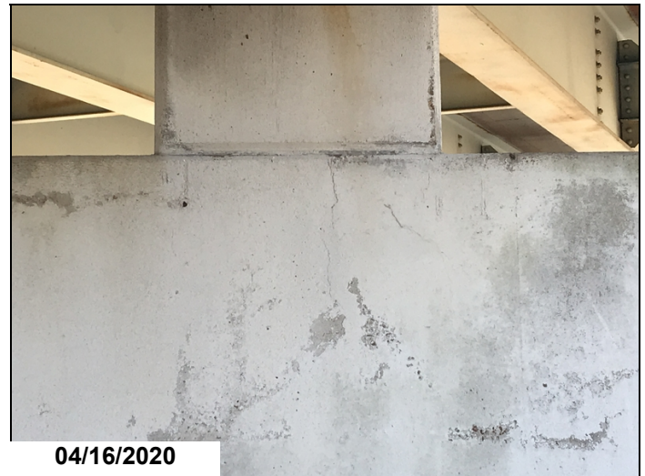
Typical vertical crack in cap under bearing riser.
