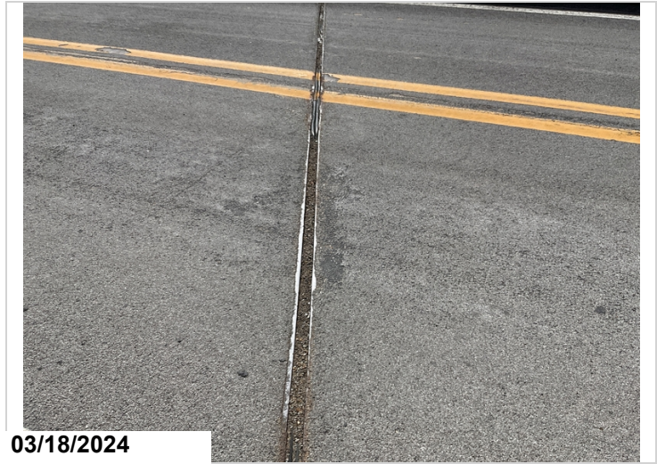
Bent 4, Compression Joint Seal: 18' of lost adhesion seal is sagging. 18LF CS3
