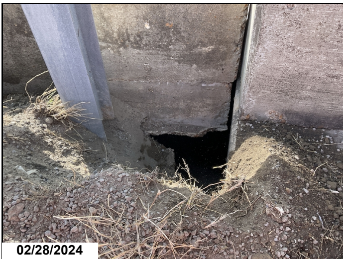
Abutment 2, Approach Roadway & Shoulder, Left: Large void 5' (depth) under roadway.
