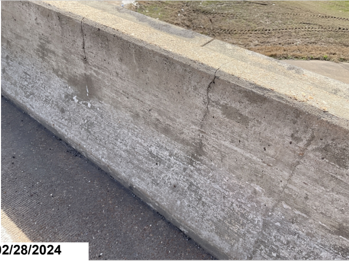
Typical bridge rail crack
