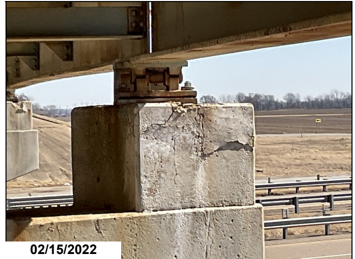
Bent #2 riser under girder #5 cracked and delaminated
