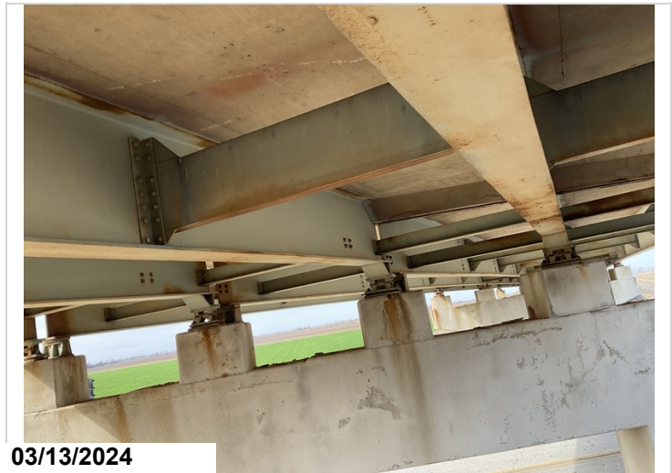
All Spans, All Girders, Full Length: Paint is discolored and oxidized with minor areas of bare steel full length. 6,445SF CS2, 6,446SF CS3, 678SF CS4
