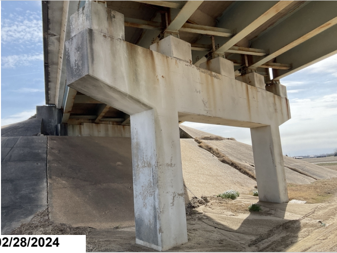
Bent 6, Pier Cap, Back, Under Girder 2: Riser has cracking at top. 1LF CS3
