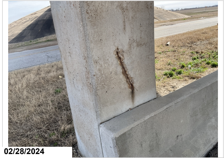
Bent 5, Column 1, Back: 3' piece of cage steel exposed due to poor concrete coverage. 1Each CS3
