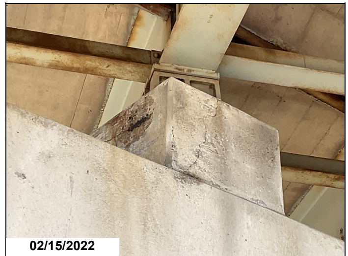
Bent #3 riser under girder #3 cracked and spalled with exposed rebar
