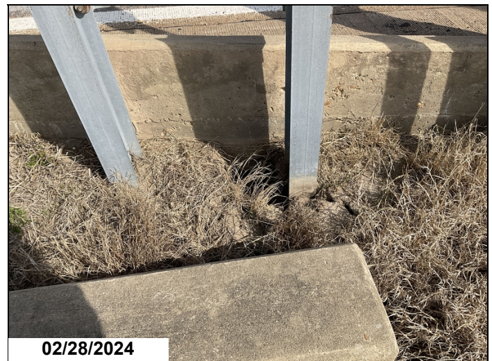
Abutment 2, Approach Roadway & Shoulder, Right: Small void under roadway.
