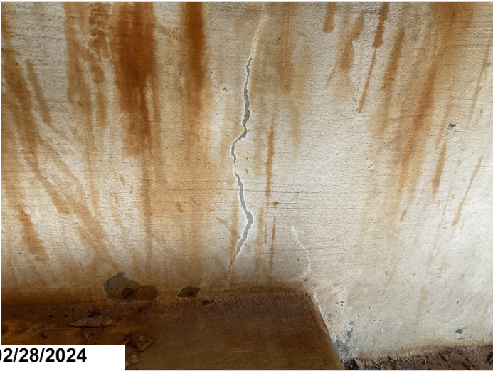
Both Abutments, Backwalls: Vertical cracks. 8LF CS2
