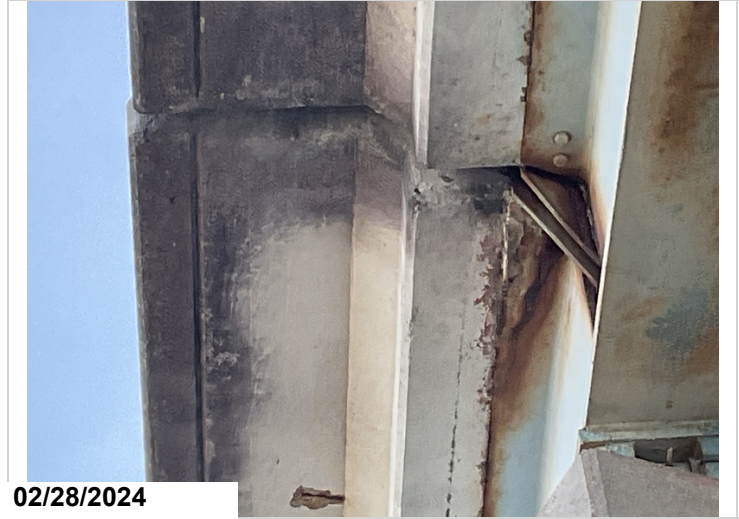
All Spans, Girders 1 & 5, All Bents, Haunch: Slight out of plane bending due to pact rust between girder and haunch.
